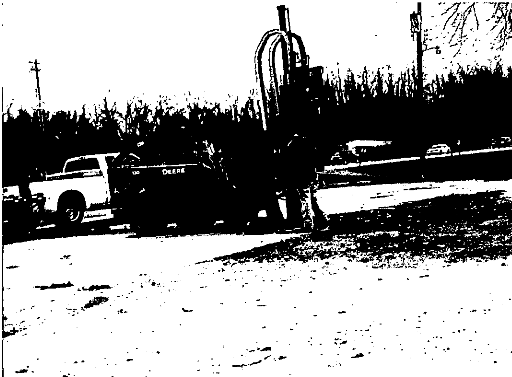
Date: 12/6/12 Time: 11:00am Direction: SE Photo by: Robert Mileur Exposure #: Comments: Conducting soil boring that will later be a MW as well.
