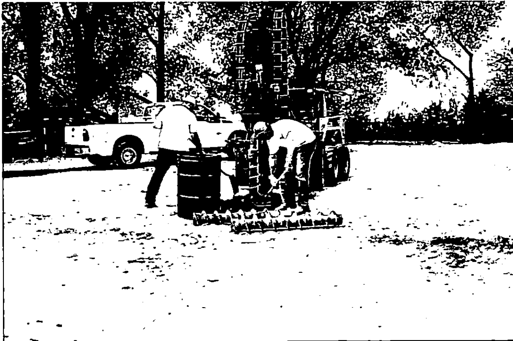
Date: 5/7/2014 Time: 10:30am Direction: Photo by: Robert Mileur Exposure #: 004 Comments: Placing augured material in drum for disposal.
