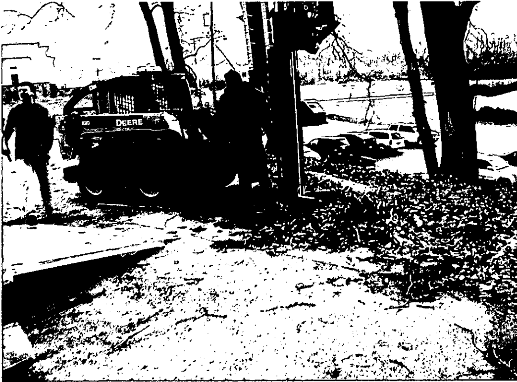
Date: 12/6/12 Time: 9:20am Direction: SE Photo by: Robert Mileur Exposure #: 001 Comments: Conducting soil boring on south end of lot.
