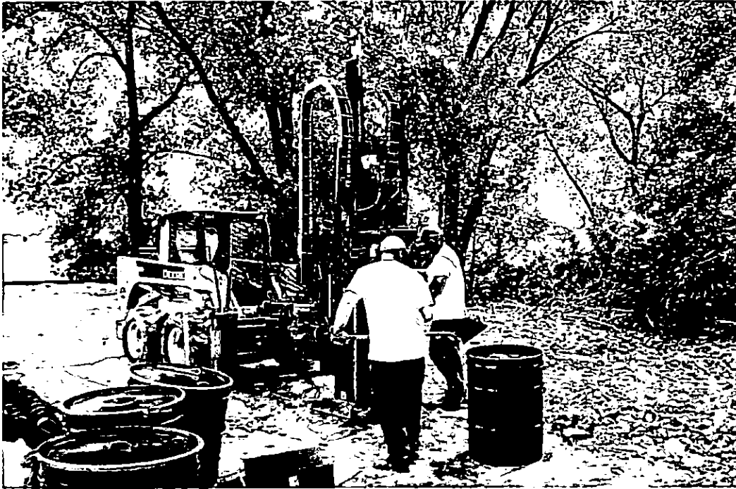
Date: 5/7/2014 Time: 2:25pm Direction: SW Photo by: Robert Mileur Exposure #: 011 Comments: Drumming tailings for MW.
